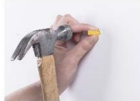
3 Use Hammer To Tuck The Plug
